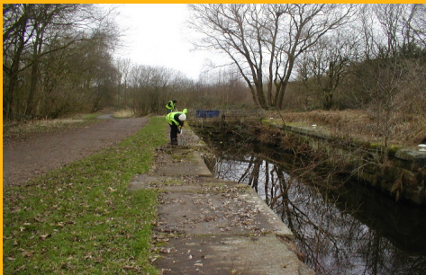
Encroaching vegetation being cleared from the lock side coping stones, before (left) and after (right)
