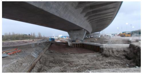
As can be seen above, one of the support pillars for the approach road lies partly within the canal bed but engineers have not only left enough vertical clearance, but also ample room for navigation along the canal, at the same time they have excavated and removed many tons of toxic materials which had accumulated on the canal bed from Widnes industries. The re-watered canal now passes below the elevated road with plenty of room.
