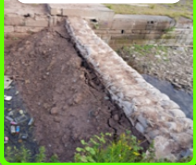
Clay bund sealing the dam
