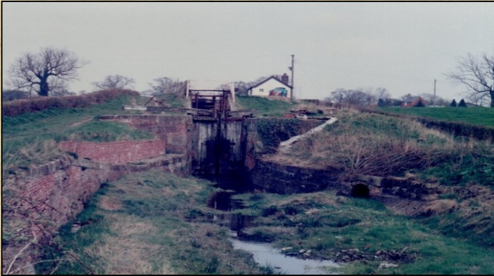
Frankton Lock before restoration
