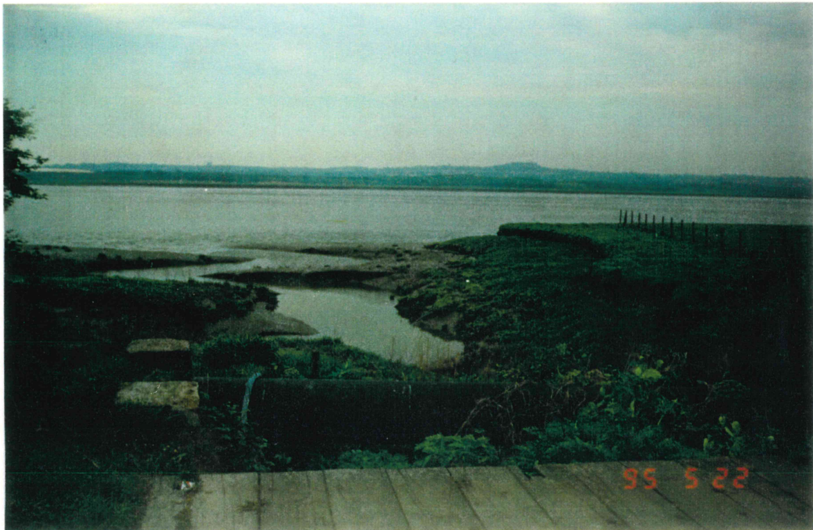
PHOTOGRAPH 1/10 - Channel From Weir to the River Mersey
