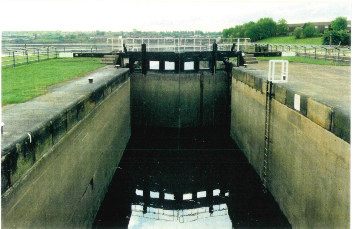
PHOTOGRAPH 0/3 - Downstream Lock Gate
