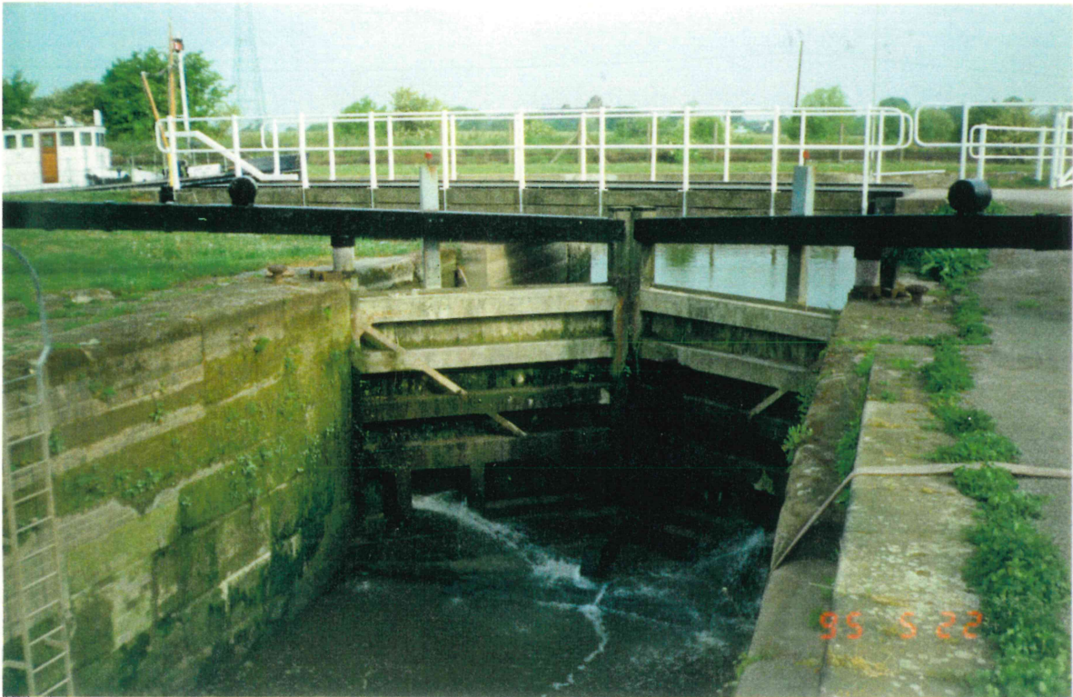
PHOTOGRAPH 1/31 - Upstream Lock Gates
