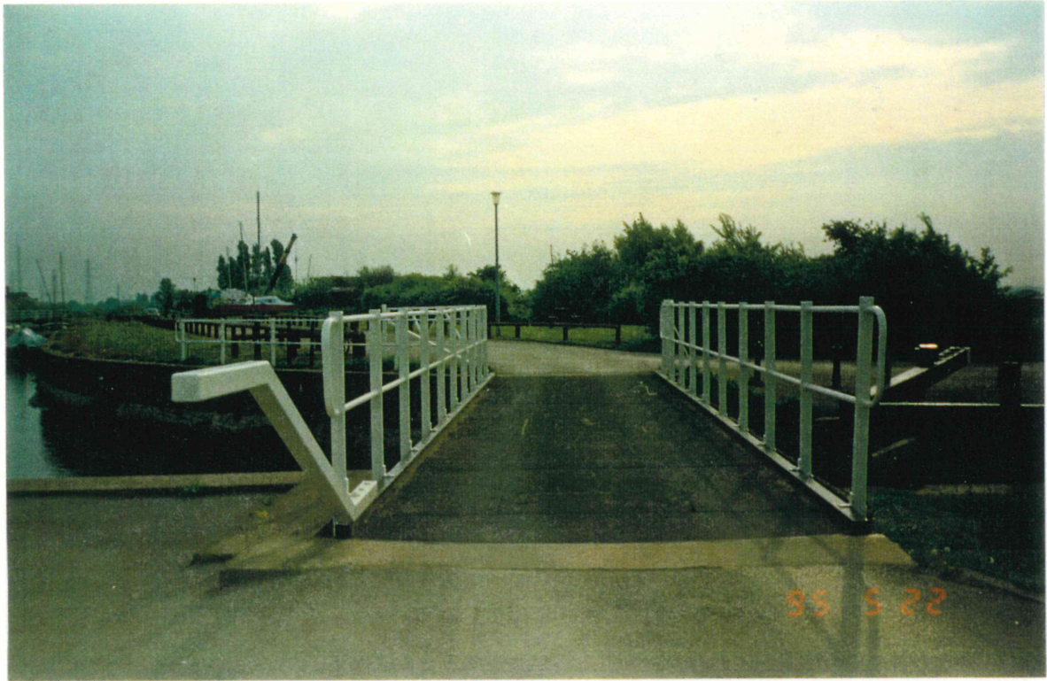
PHOTOGRAPH 1/28 - General Elevation of Carriageway
