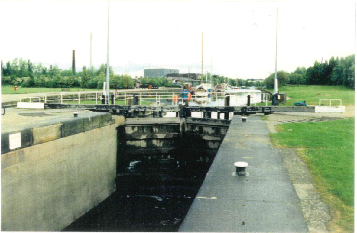
PHOTOGRAPH 0/1 - Upstream Lock Gate
