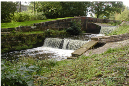
Old Double Locks before the repairs
