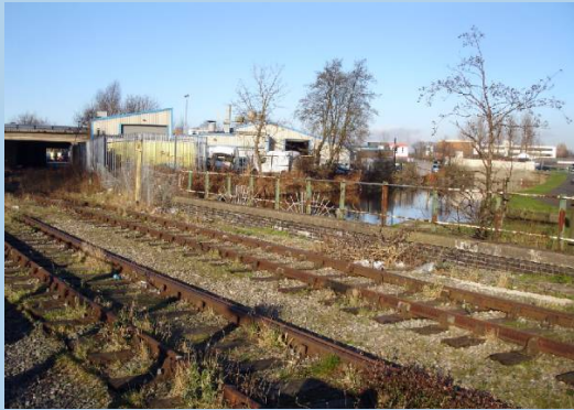
Site of former swing bridge
