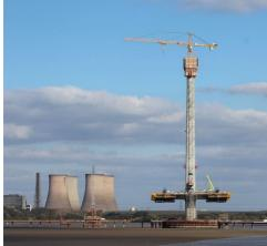
The Mersey Gateway's south bridge pylon is now complete, *(left)* marking the project's highest point in the River Mersey estuary. The south pylon stands at an impressive 125 metres high, while the north pylon measures 110 metres. The smaller central pylon, due to be finished in November, will be 80m. high.
